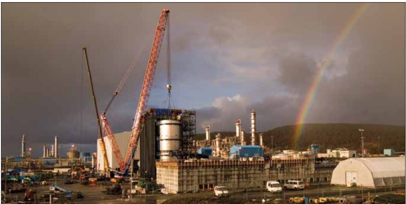
The Eurogas-Marcogaz LCA covers all steps of the natural gas chain – a gas-fired combined cycle power plant under construction in Kårstø, Norway.
