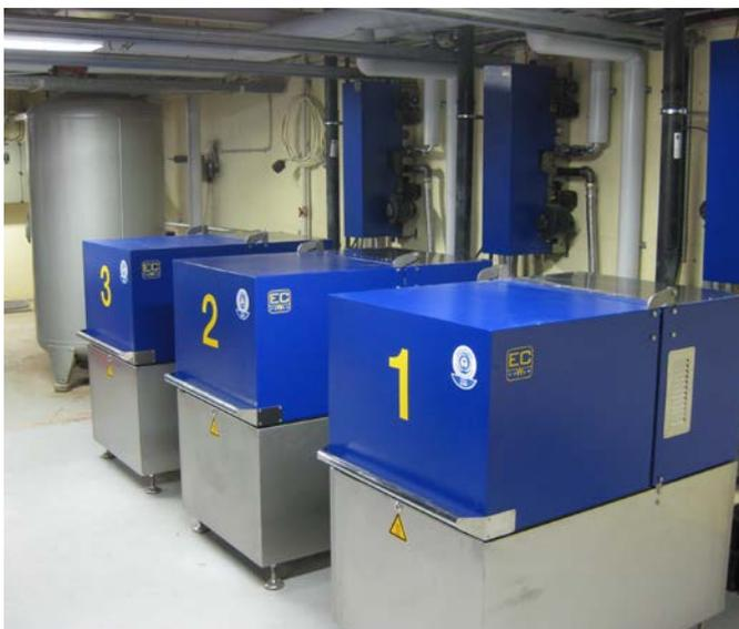
Figure 2. An installation with three cogeneration units (20 kWe each). This installation also includes a heat pump (not shown in the picture) and four storage tanks with a total volume of 3500 litres.
